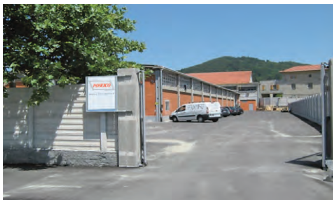
New facility (May 2011) Power Rectifiers and Converters; Power assemblies; Devices for Traction Substations via Milite Ignoto 11 Busalla (20 km from Genova) Italy
