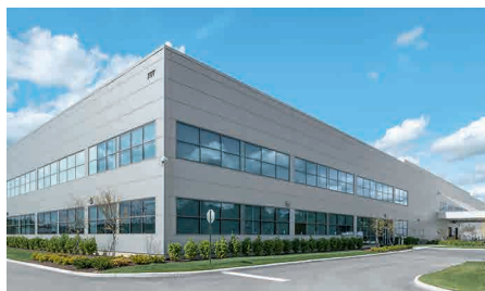
A central position in the Midwest: Mason in Ohio, USA. 70% of customers are located within a radius of 1,000 kilometres.
