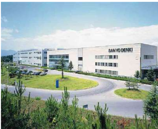
FUJIYAMA WORKS, Ueda (Japan) Built 1990, Floor Space 82,821 sq.m, ISO 14001
