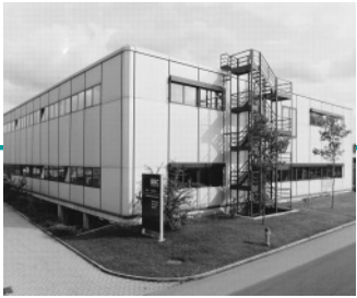
1981 Inauguration of BBC high power semiconductor factory in Lenzburg, Switzerland
